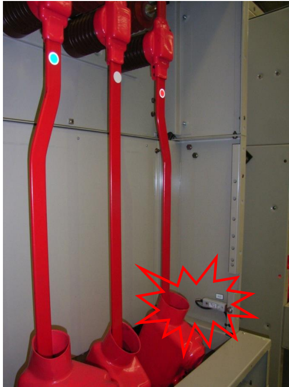
Sensor placement inside cable termination chamber
