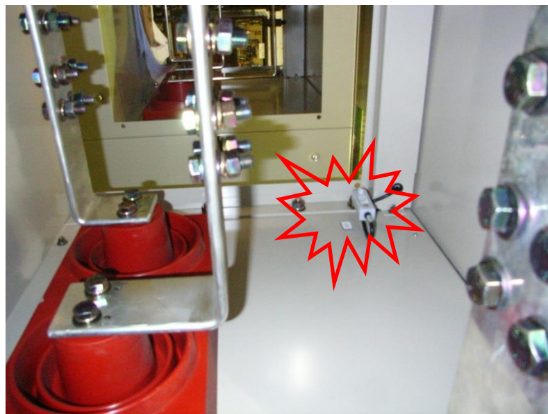
Sensor placement inside busbar chamber
