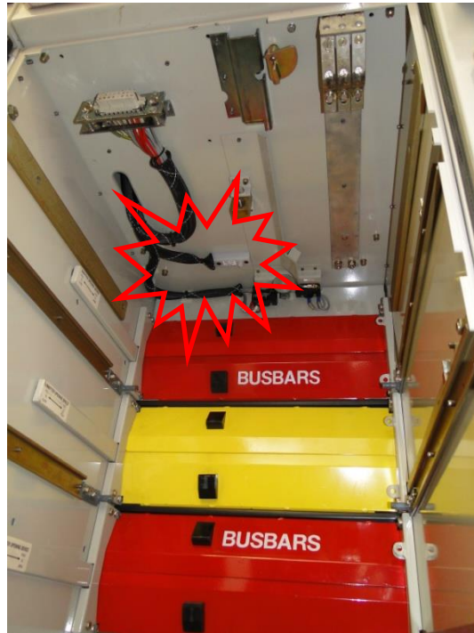
Sensor placement inside CB racking chamber
