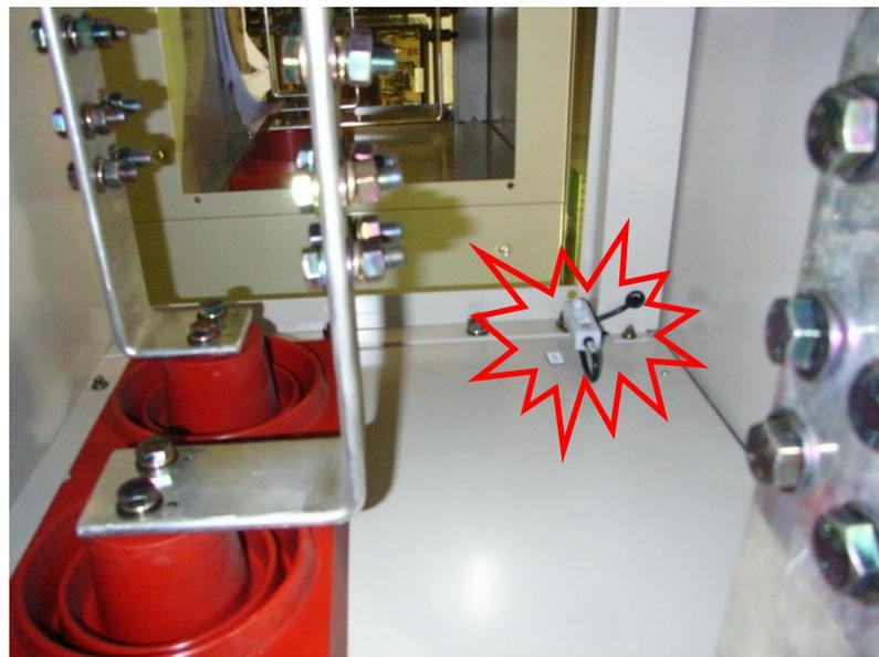
Sensor placement inside busbar chamber
