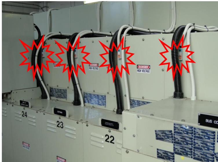
Sensor placement for switchgear Busbar coverage (External through Hole Detector)
