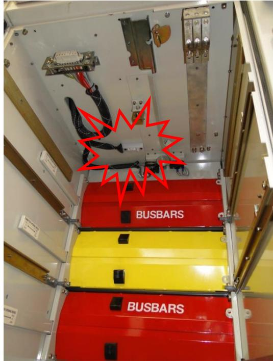
Sensor placement inside CB racking chamber
