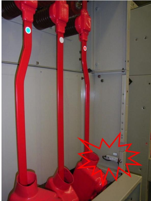
Sensor placement inside cable termination chamber
